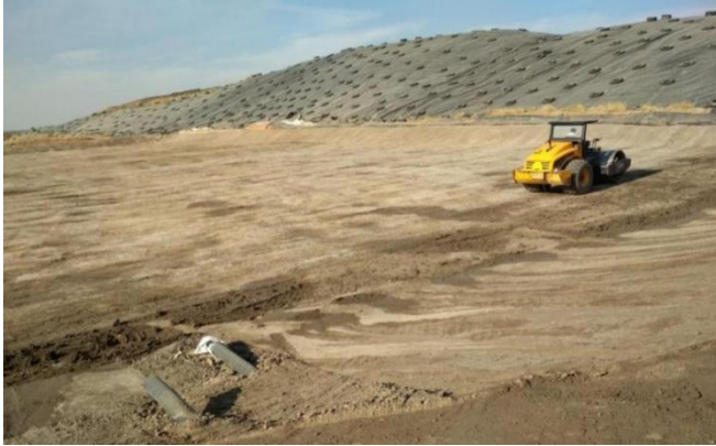
Figure 12.6: Clay laying at base
