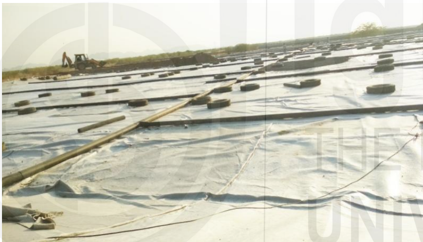
Figure 12.11: Leachate collection pipes (header 200mm + lateral 160mm)
