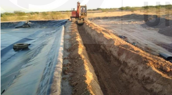
Figure 12.7: Anchor trench opening
