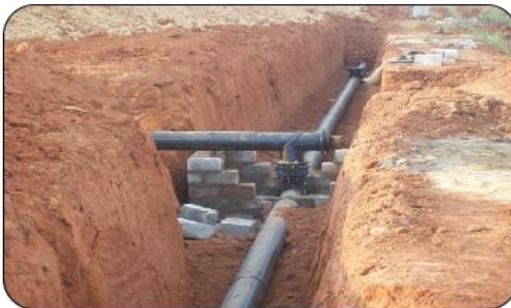
Figure 12.11: Leachate collection pipes (header 200mm + lateral 160mm)
