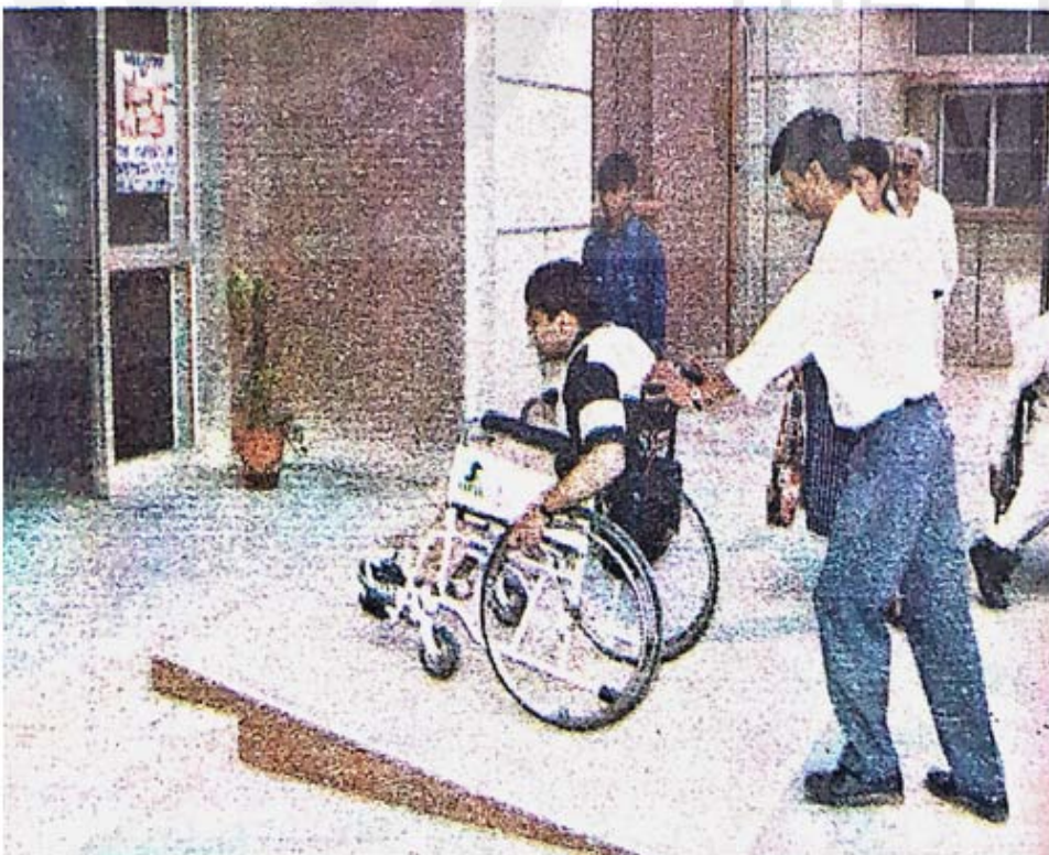
Fig 1. A ramp over the stairs at the entrance makes the building accessible to wheelchair users
