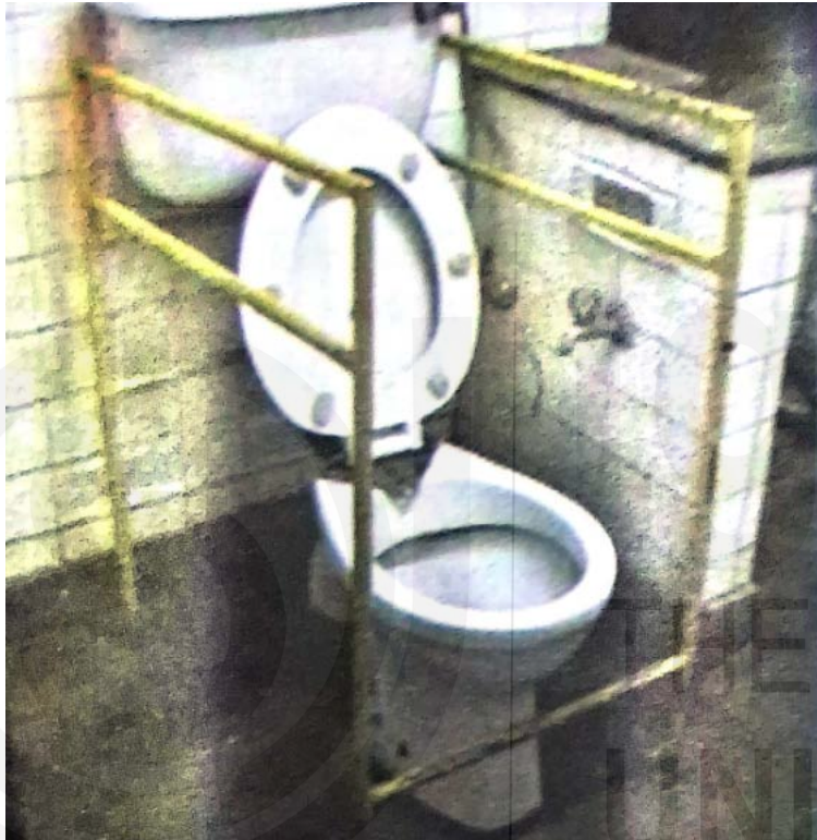
Fig. 6: Hand rails around the toilet seat help the person with disability to use it while standing
