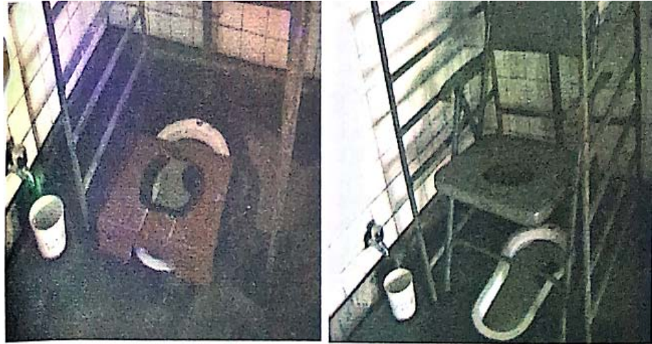
Figs. 7(a) & (b): Chairs and stools of varying heights can be placed over the Indian style toilet to enable the person to use it.
