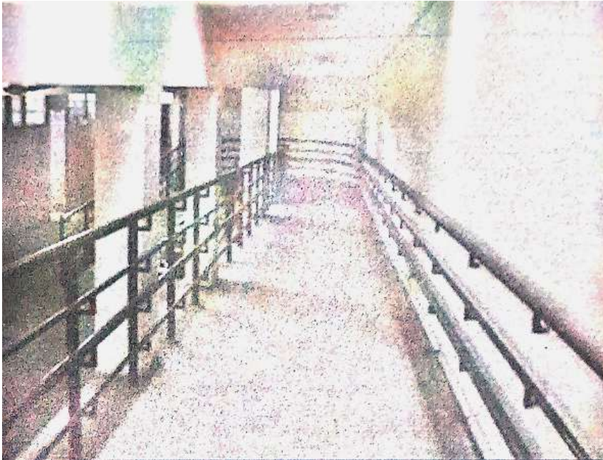
Fig. 3: A ramp with a gradual slope and hand rails at two levels
